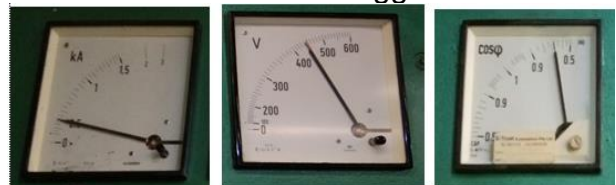
Gambar 2.2 Parameter generator (Amperemeter, Voltmeter, Cos phi meter)
